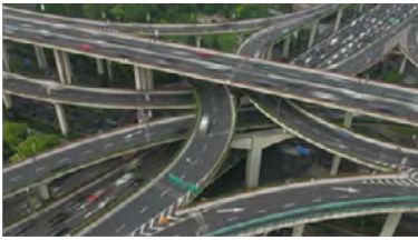
Multilevel highway interchanges pose a problem to satellite positioning: which road am I on? 3D Dead Reckoning solves this dilemma
