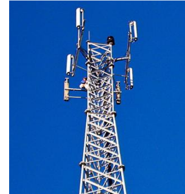
Cellular base station, using a GNSS receiver for synchronization
