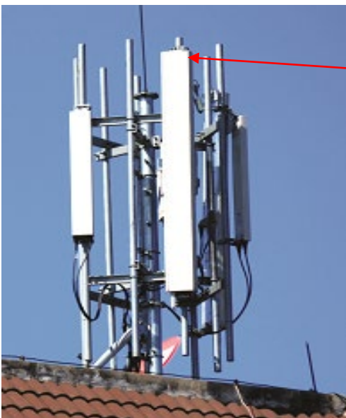
Figure 14: Cellular base station antenna pointing application.
