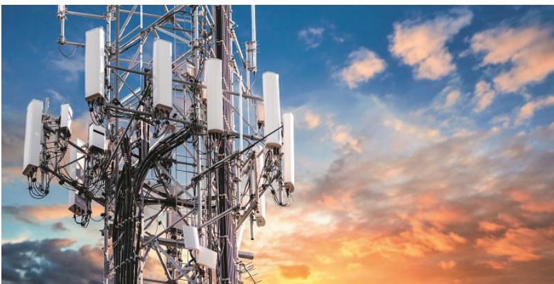
Figure 8: Antenna pointing systems – base and rover on a single-cell antenna panel
